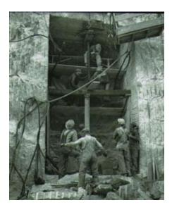
Construction of the hall took place between July 1938 and July 1939, when a 70-foot tunnel was blasted into the mountain. It remains very rough cut, and tapers to a point at the back. Work halted in 1939 when Congress directed that construction should be executed only on the faces. With Borglum's death in 1941 and American involvement in World War II, all work on the memorial came to a close on October 31, 1941.
